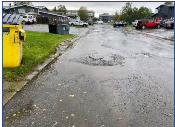
Curb heaving and pavement failure along 75 th Avenue
